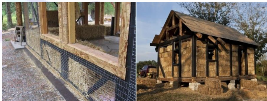
Figure 1: Different stages of straw bale house construction (Morrison)
